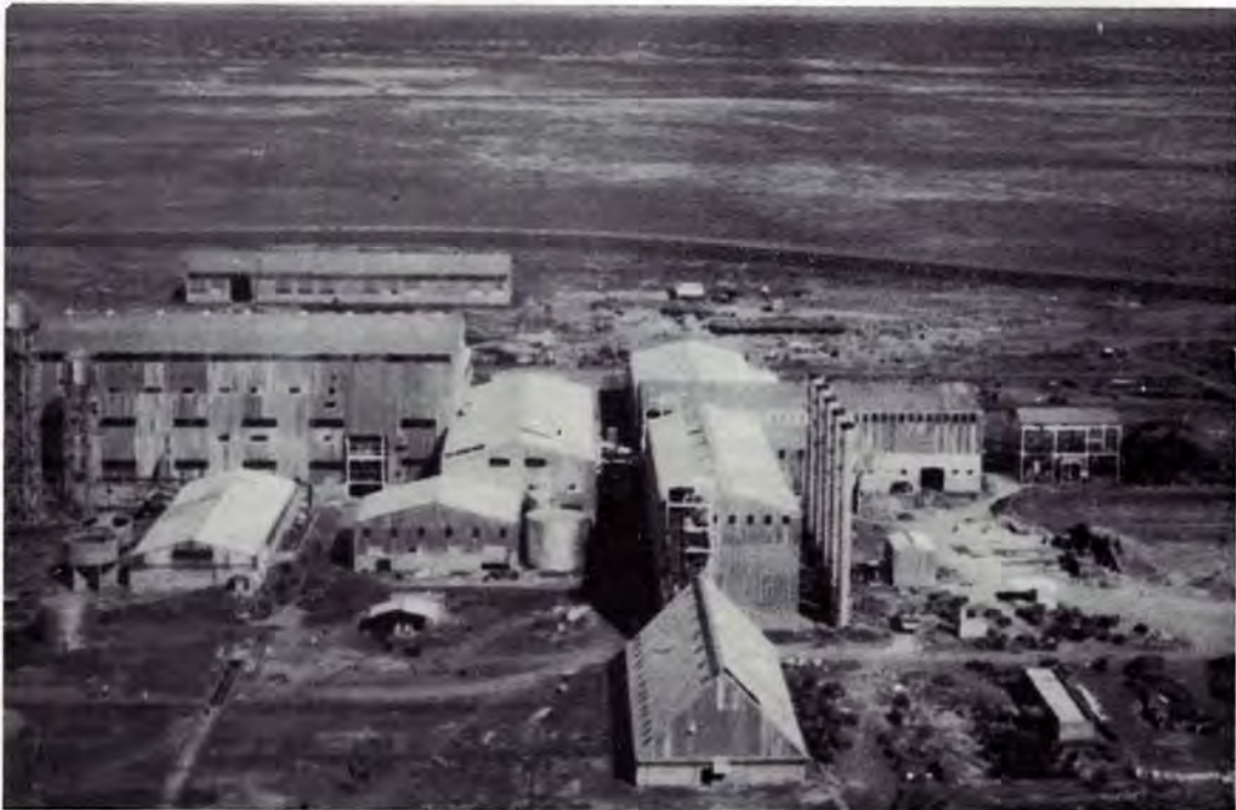
An aerial view of the Asalaya total energy concept sugar refinery.
